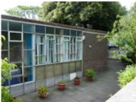
School hall on corner of Ashmount Road and Hornsey Lane.
