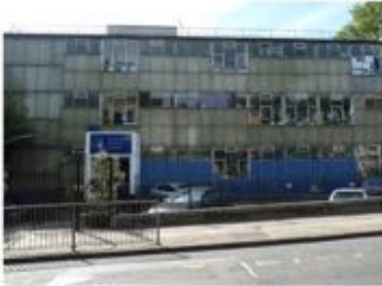
Front elevation of junior school building facing Hornsey Lane
