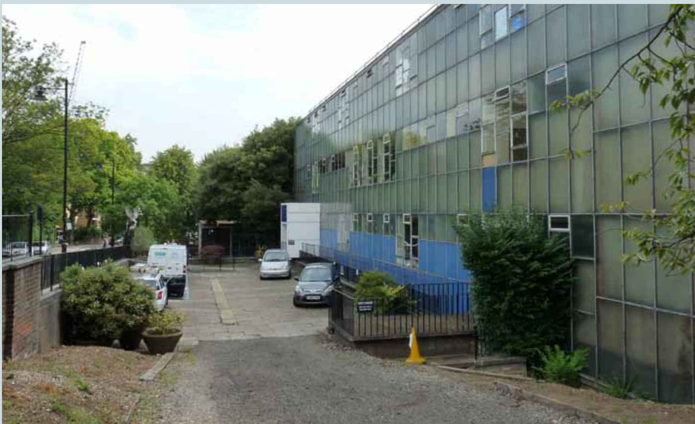
The front of the school and space between the school and Hornsey Lane
